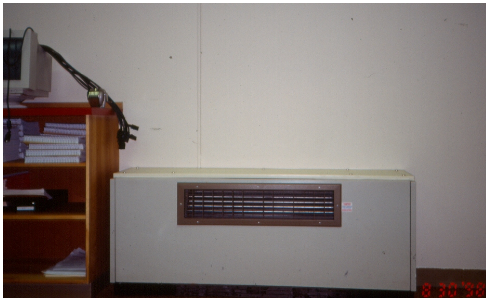
Figure 2. Console heat pump.
