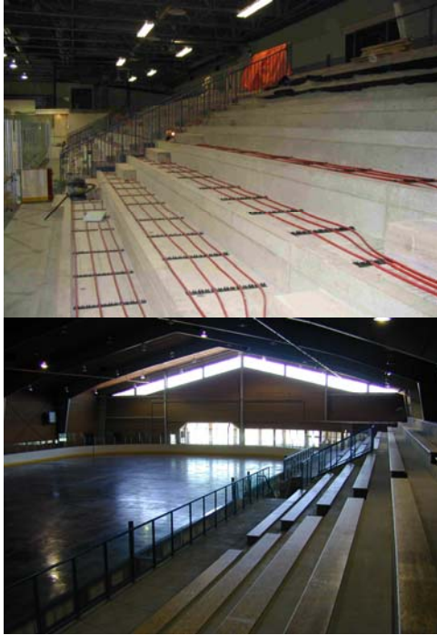
Figure 3. Much of the building, including the spectator seating, is heated with a radiant floor heat system. The warm floor dries snow that is tracked from outside into the building and reduces the opportunity for mildew growth in the change rooms.
