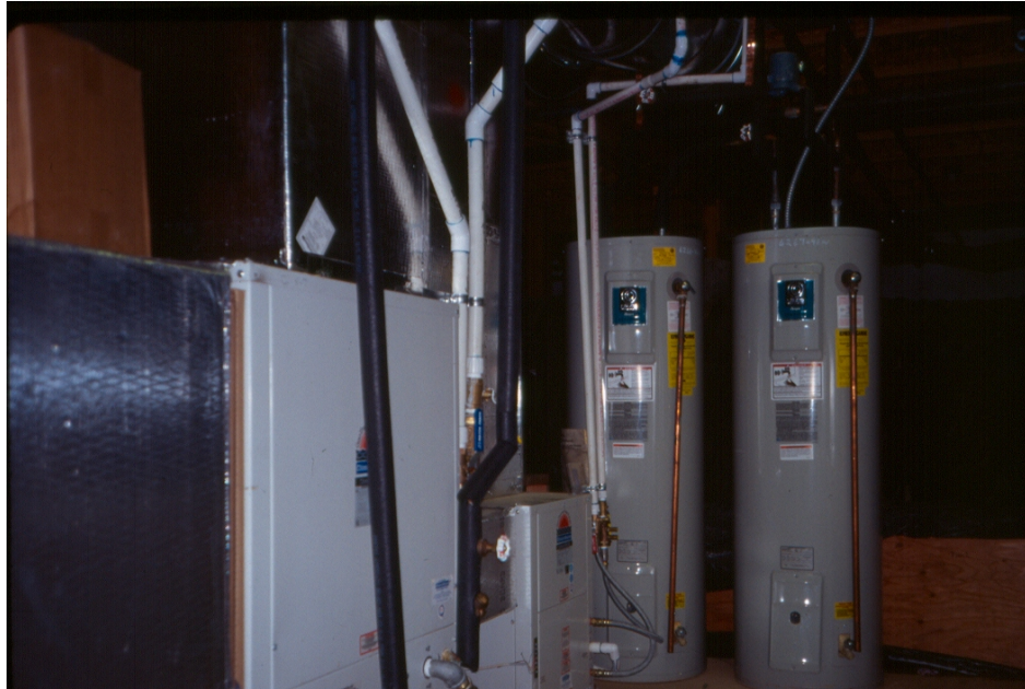
Figure 3. Water to water heat pump.
