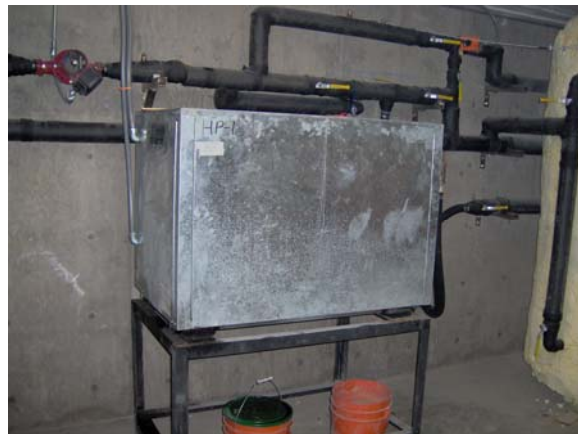
Figure 3. Photograph of the 15 ton water-water heat pump serving the entire building. Note the storage tank on the right.
