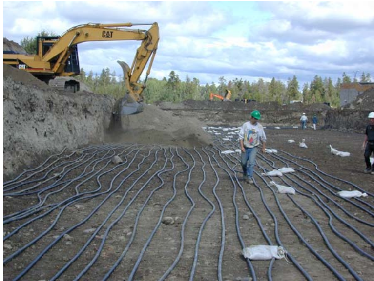
Figure 3. Much of the building, including the spectator seating, is heated with a radiant floor heat system. The warm floor dries snow that is tracked from outside into the building and reduces the opportunity for mildew growth in the change rooms.
