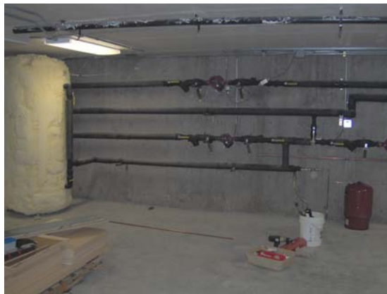
Figure 3. Photograph of the 15 ton water-water heat pump serving the entire building. Note the storage tank on the right.
